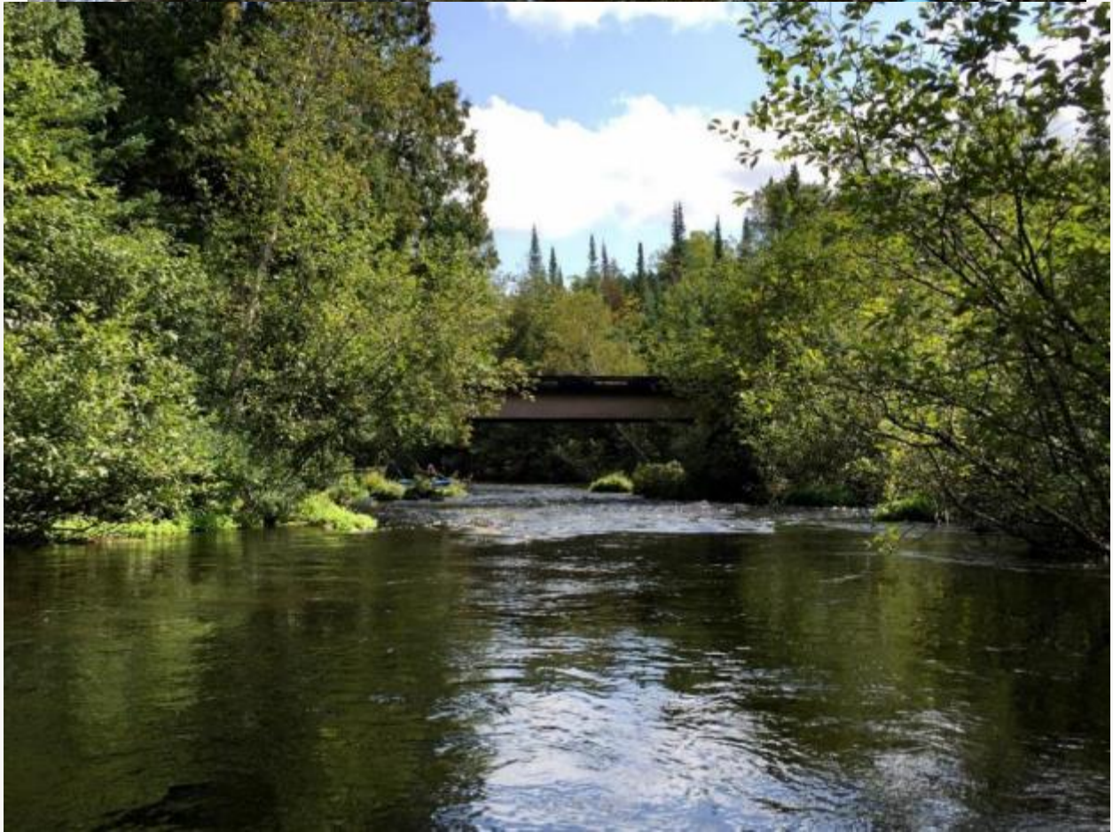
Cedar Island Road Bridge
